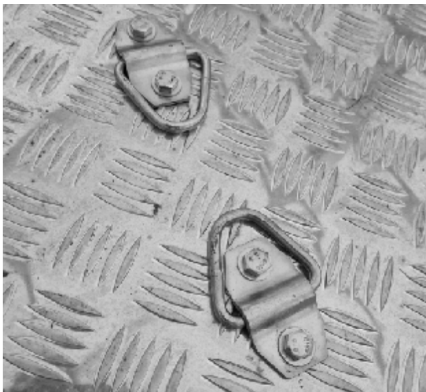
Figure 4.15 – Fall Restraint Points
